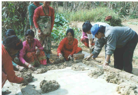
Figura 4: Colocando ladrillos. Foto: E. Judge / Practical Action.
